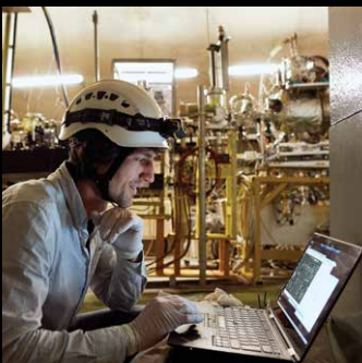
Redundant and Remote Networks
